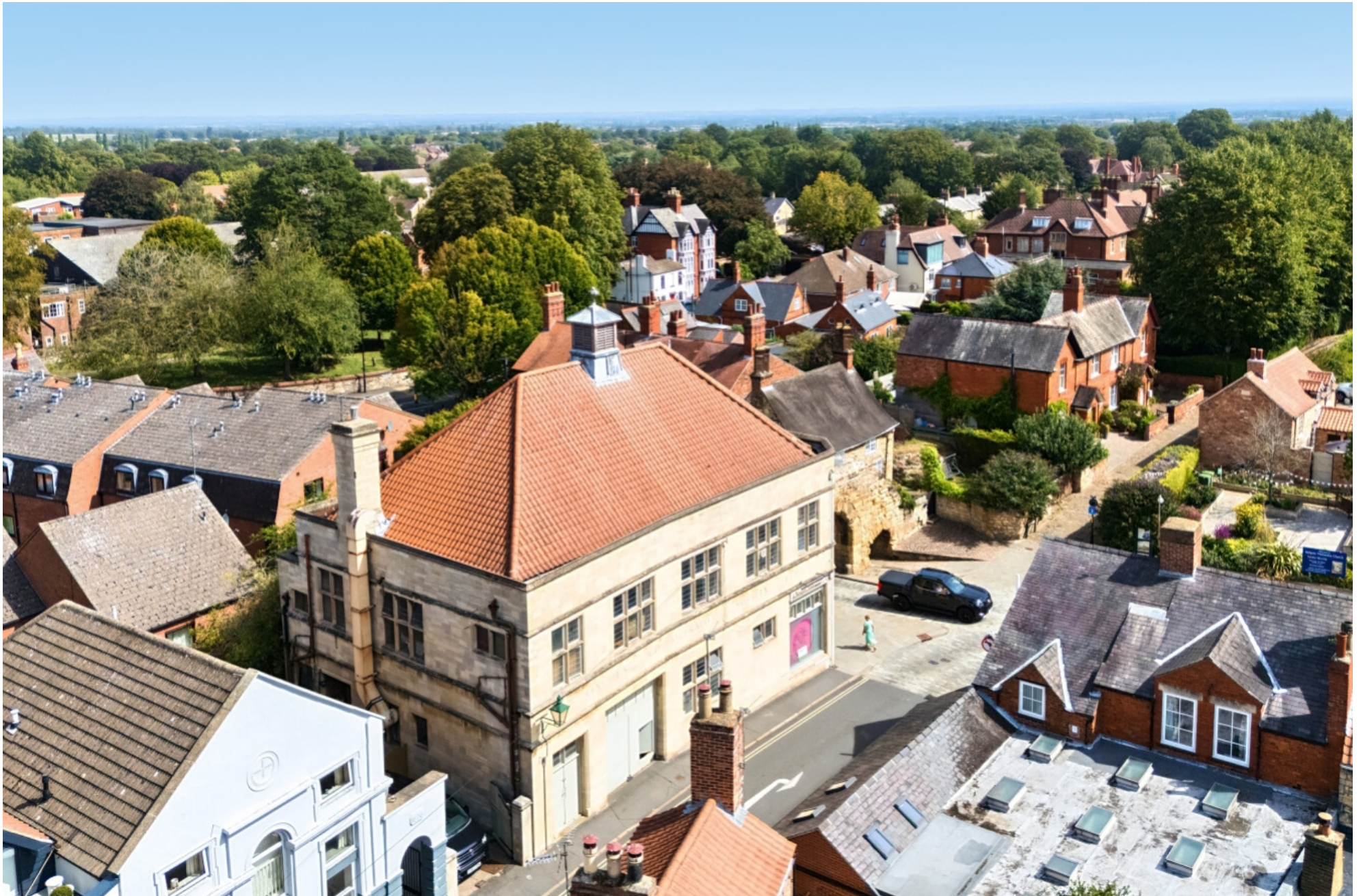
Newport Arch, 50 Bailgate, Lincoln, Lincolnshire, LN1 3AP
