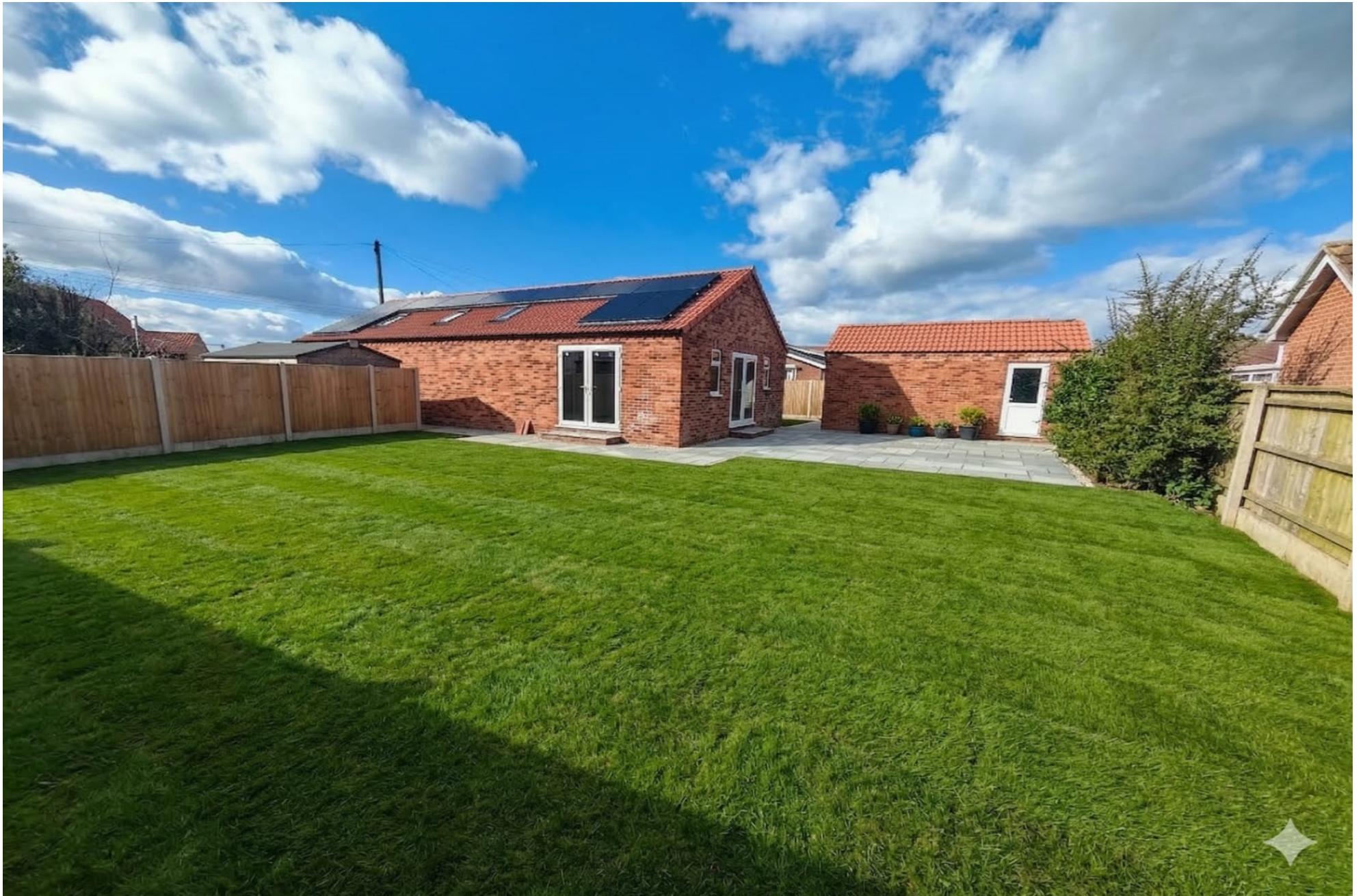
New Build Adjacent to The Oak, South Street, Swineshead, Boston, Lincolnshire, PE20 3JD
