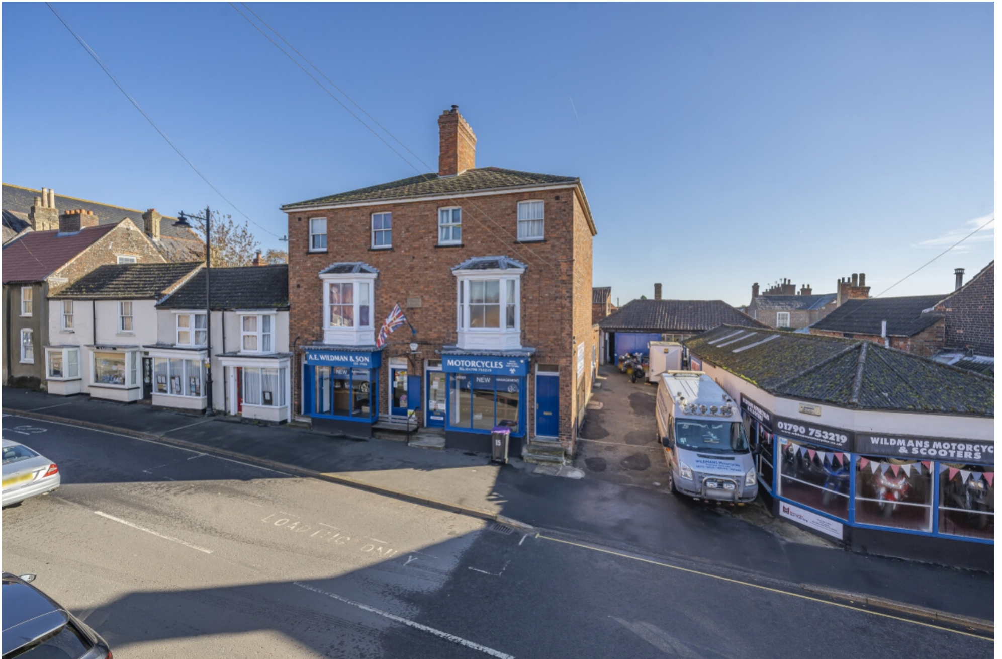
Shop & Flats , 11-15 Halton Road, Spilsby, Lincolnshire, PE23 5JZ
